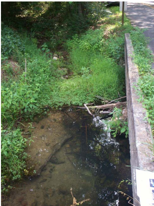
View upstream at the Autry Road crossing.
