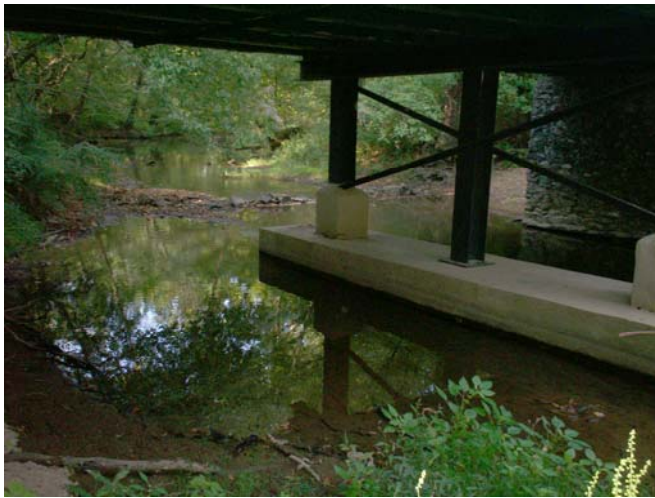
View downstream under the Minshew Road bridge crossing
