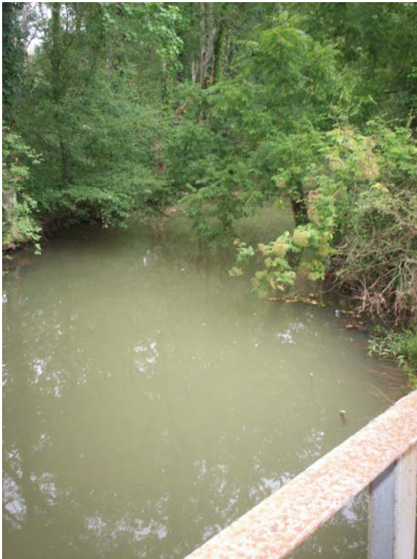
Gaines Loop crossing view downstream.
