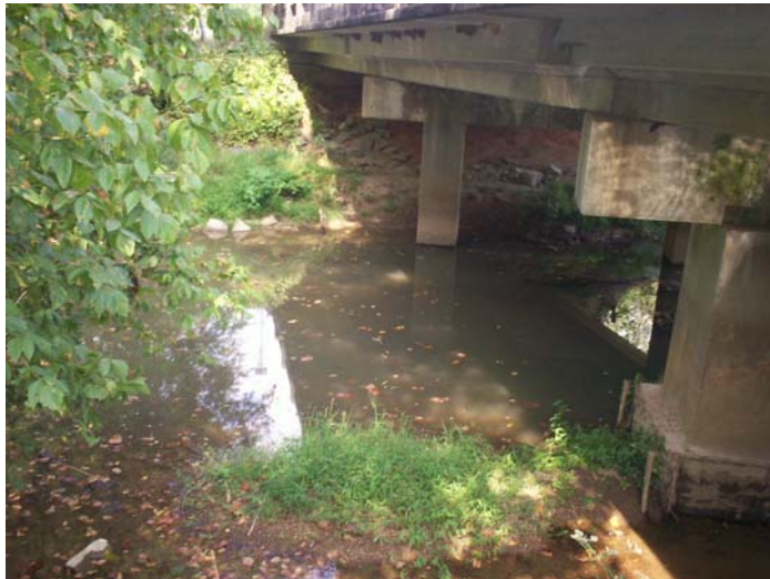
View below bridge
