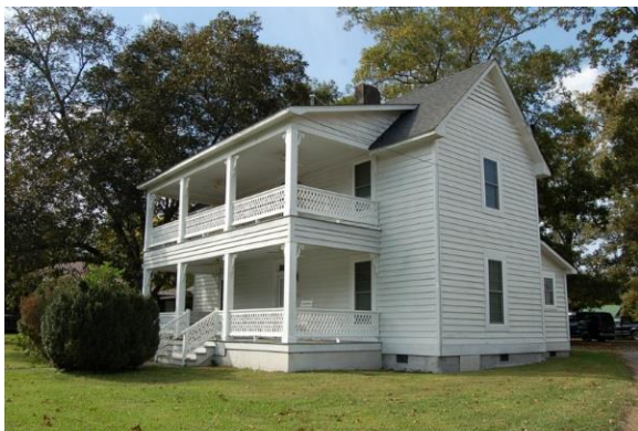
FIGURE 24. TOM BAGBY HOUSE, WOLFE STREET
