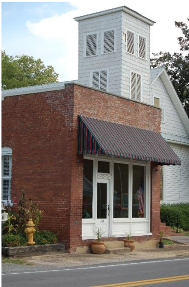
FIGURE 1. TOWN CLERK'S OFFICE, WOLFE STREET
