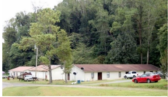
FIGURE 11. MULTI-FAMILY RESIDENTIAL HOUSING ON MOUNT OLIVET DRIVE
