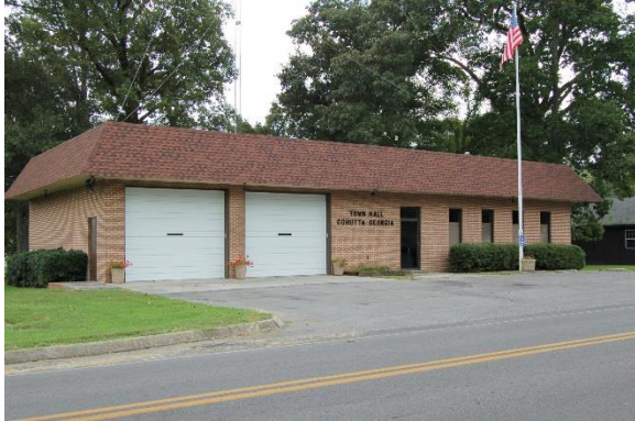
FIGURE 20. COHUTTA'S TOWN HALL, RED CLAY ROAD
