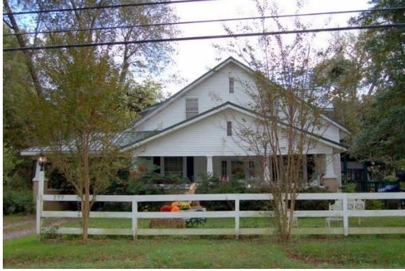
FIGURE 27. JOHN H. SHUGART HOUSE, WOLFE STREET
