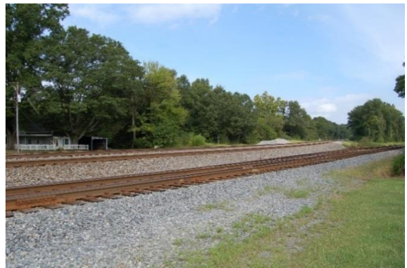
FIGURE 15. NORFOLK SOUTHERN RAIL LINES GOING NORTH OUT OF COHUTTA
