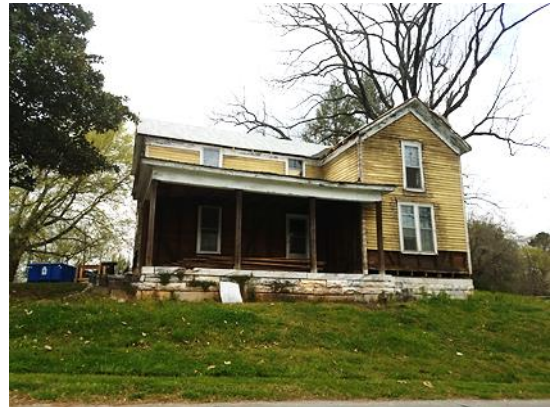
Figure 88: Historic single family detached residence under renovation in Nelson. Note the use of marble blocks for the foundation, a common practice within the traditional neighborhood.
