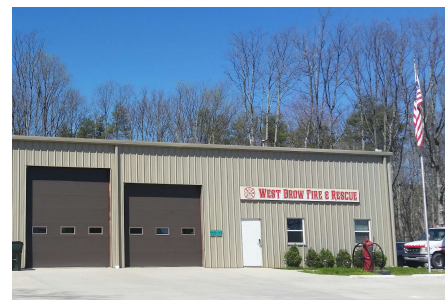
Figure 59. West Brow Fire Station.
