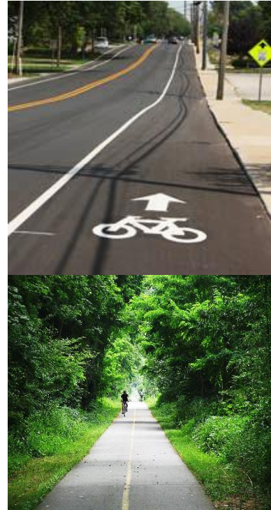
Examples of various bike lane designs that could be incorporated throughout Whitfield County for alternative transportation and recreation opportunities
