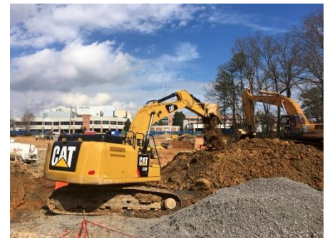
Construction of the newest addition to Hamilton Medical Center, The People's Cancer Institute
