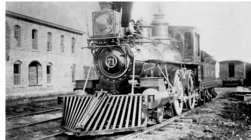
Rail freight and transportation has played a significant role throughout Whitfield County since before the Civil War
