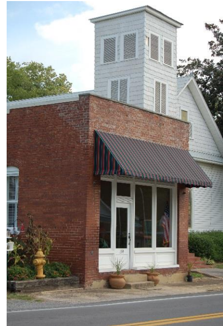
Previously utilized as the Town Clerk's Office, this building is now home to a gourmet ice cream parlor in the town center
