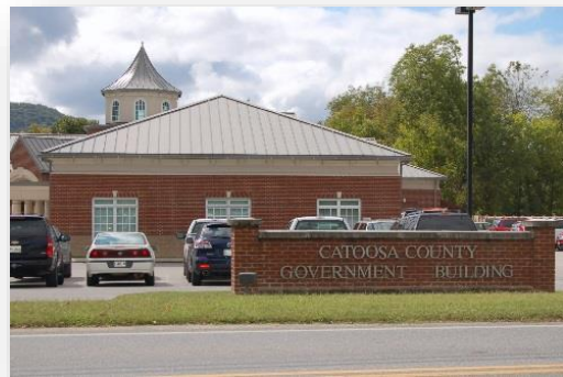
Figure 6. Catoosa County Government Building, Ringgold.
