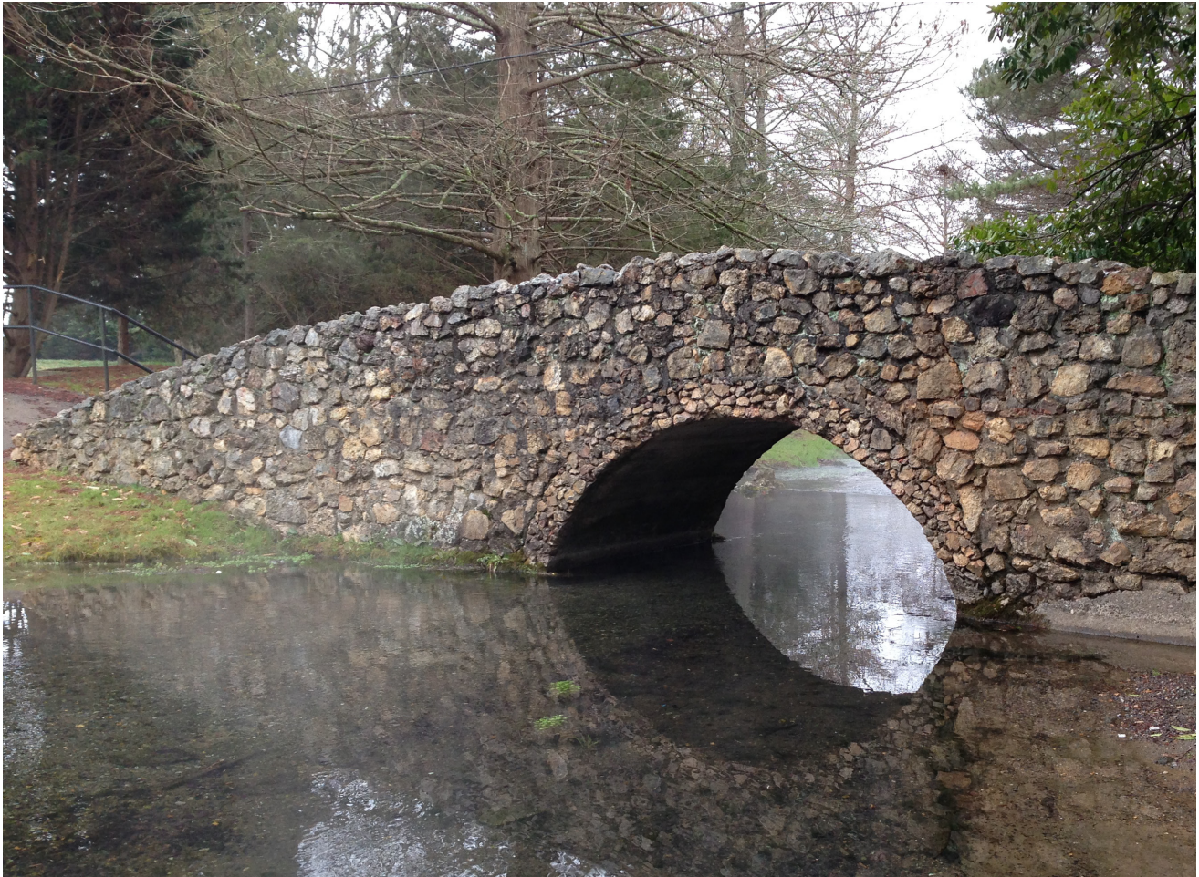
Stone bridge at Big Spring Park in Cedartown
