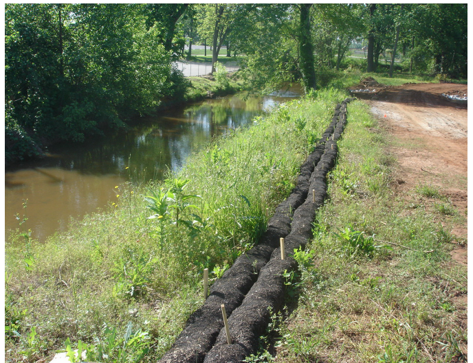
Example of a silt sock controlling drainage along a riparian trail corridor
