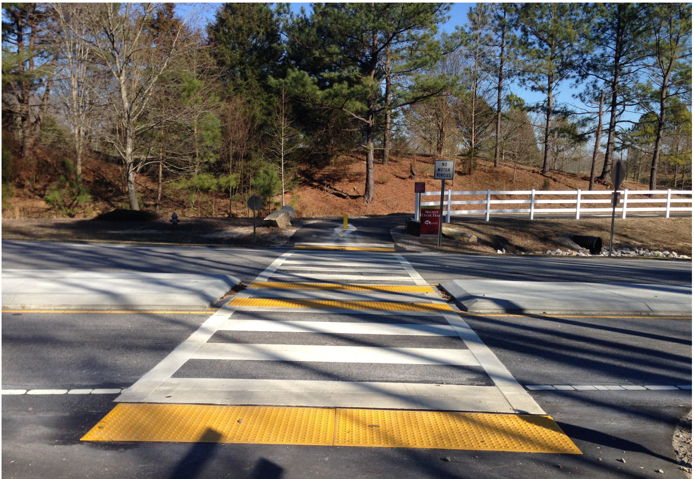
At-grade roadway intersection
