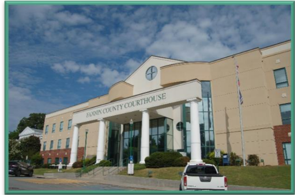
Fannin County Courthouse in Blue Ridge
