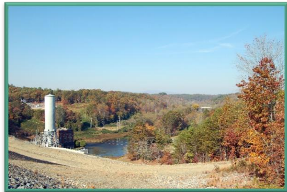
TVA Powerhouse below Blue Ridge Dam
