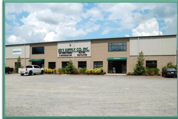
Fannin County Economic Dev. Authority spec building off SR 5
