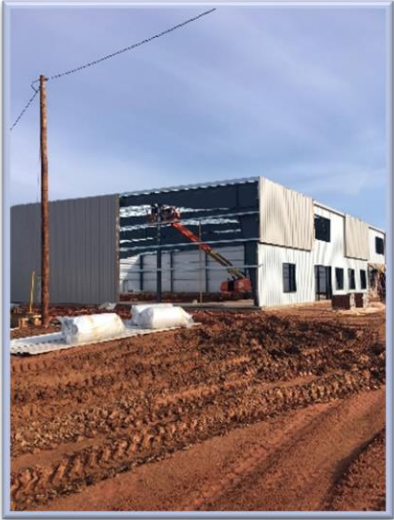
Spec Building for industry under construction on SR 5
