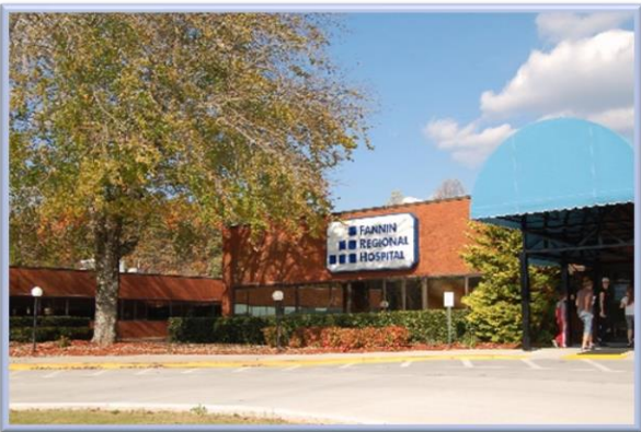
Fannin Regional Hospital on SR 5
