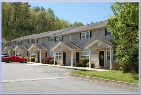
Apartments off of Mineral Springs Road in Fannin County
