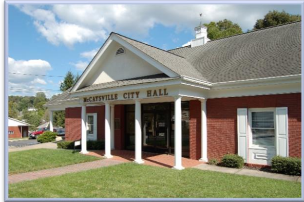
Figure 16. McCaysville City Hall
