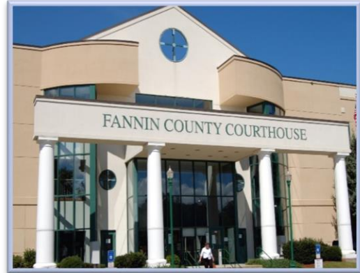
Figure 14. Fannin County Courthouse, built in 2004
