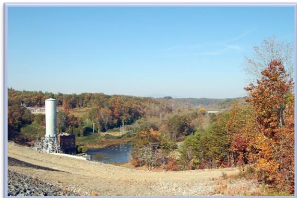
TVA Powerhouse below Blue Ridge Dam
