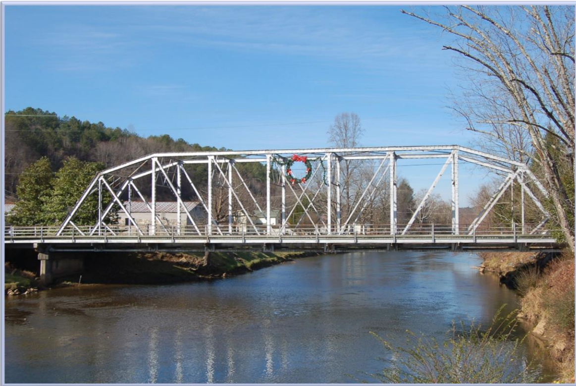
Figure 13. Steel Bridge over the Toccoa River at McCaysville
