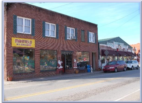
Stores across from the depot, Toccoa Ave., McCaysville
