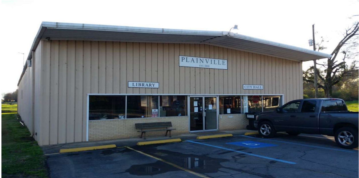
Plainville City Hall, Earl Street, Plainville.
