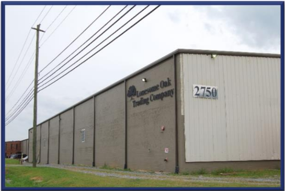
Lonesome Oak Trading Company floorcovering plant in Eton
