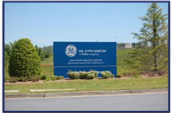
New General Electric Distribution Center, US 411
