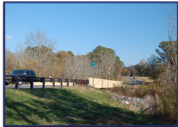
Bridge on SR 52 over Town Creek at Vann House
