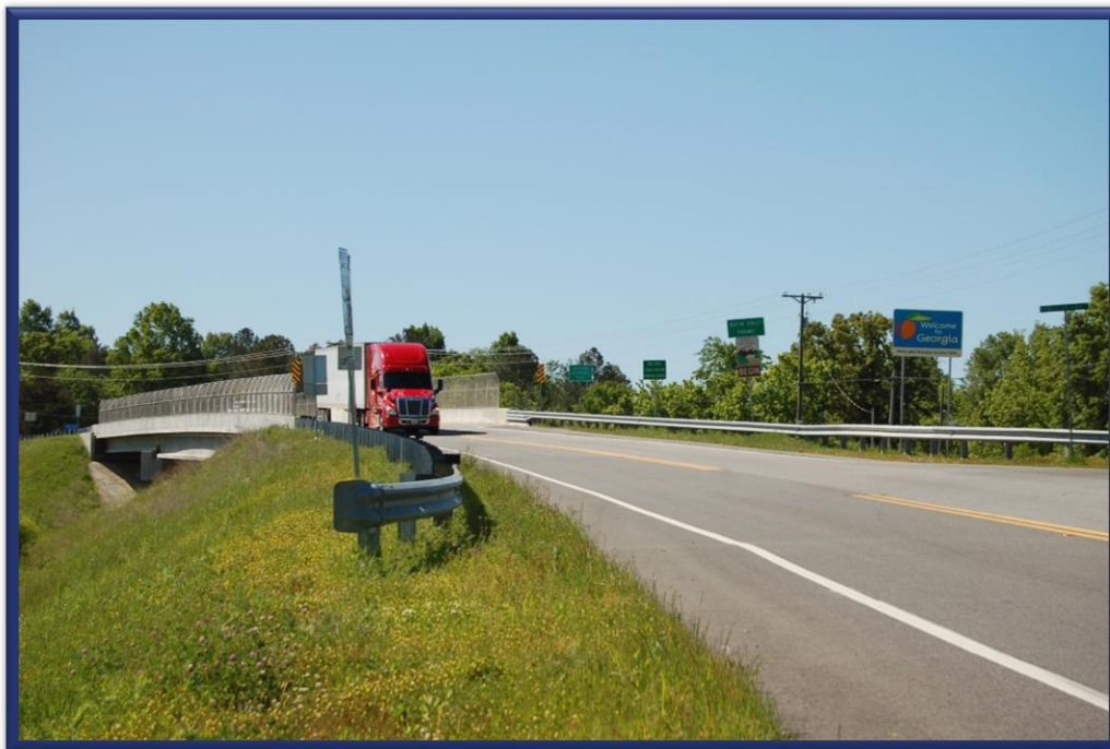
Newly completed bridge on US 411 over railroad track in Tennega
