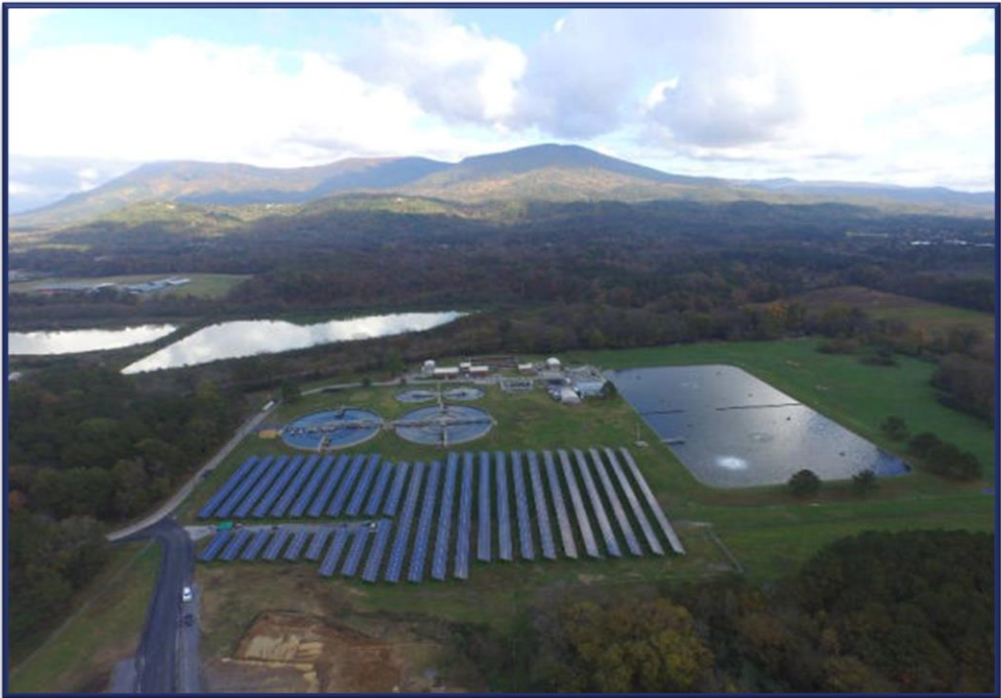
Solar Array powering the Chatsworth Waterworks Judson Vick's Wastewater Treatment Plant
