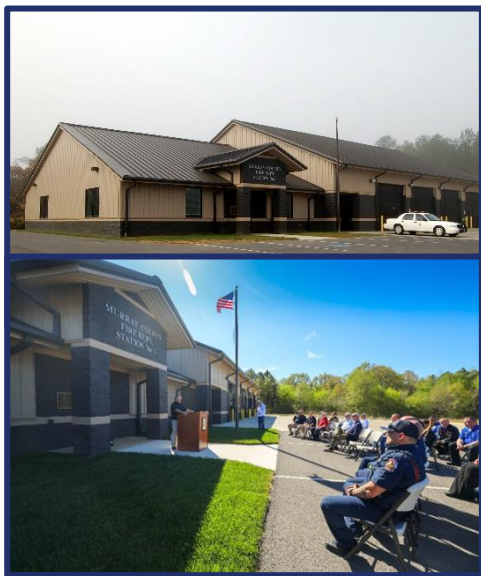
Fire Station 1 on SR 225. Lower photo by Jay Choate
