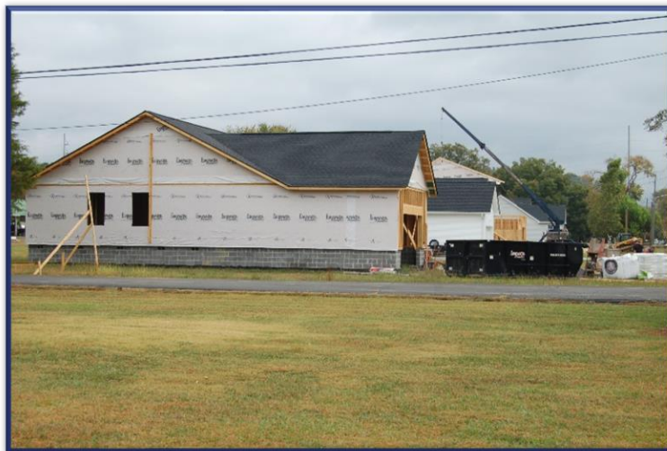
Housing construction in Eton
