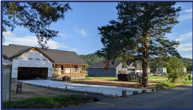
New single family housing construction in Eton
