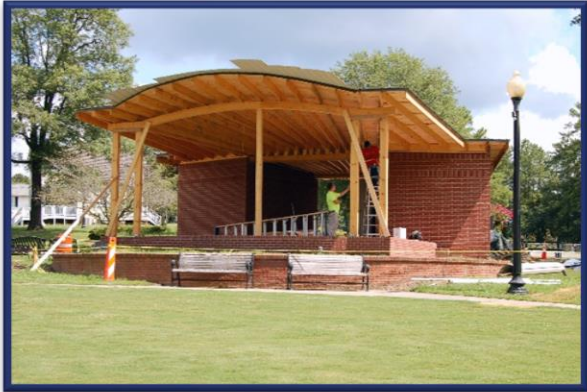
Chatsworth City Park stage under construction
