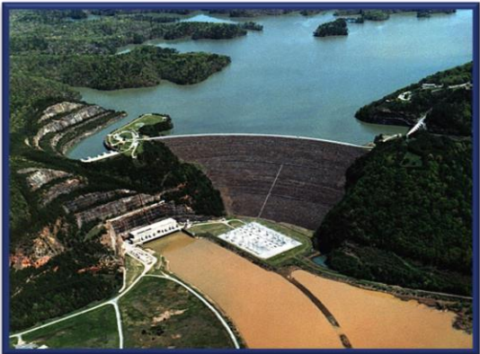
Carters Dam. Photo US Army Corp Engineers
