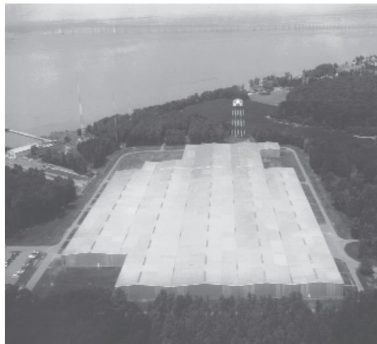
The Chesapeake Bay Model is contained in this warehouse, on Kent Island, Maryland. The Chesapeake Bay Bridge is in the background. U.S. Army Corps of Engineers Waterways Experiment Station photo
