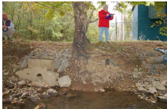
9. Shannon water intake left bank
