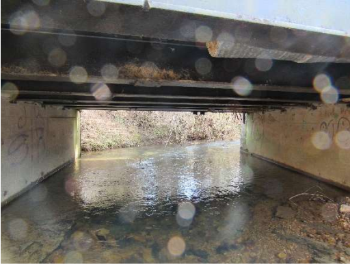
27. Buttrum Road Bridge tributary looking upstream
