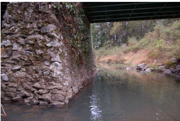
3. Bell's Ferry Road Bridge site looking downstream
