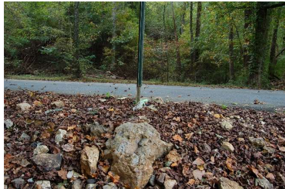
25. Autry Road Bridge left bank
