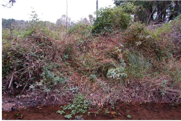
19. Plainville Road Bridge right bank
