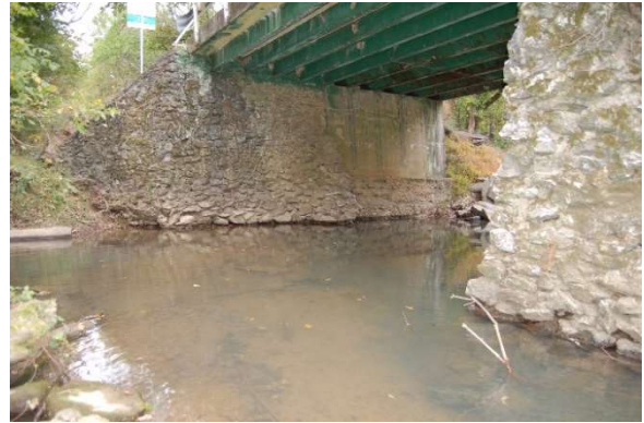
2. Bell's Ferry Road Bridge site looking at right bank
