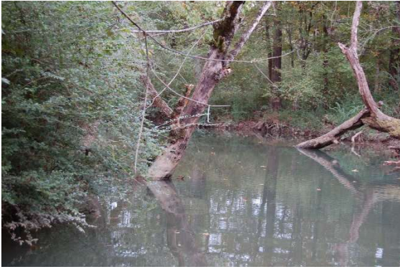
14. Gaines Loop Road Bridge looking upstream
