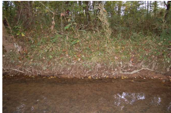
7. Shannon Water intake right bank
