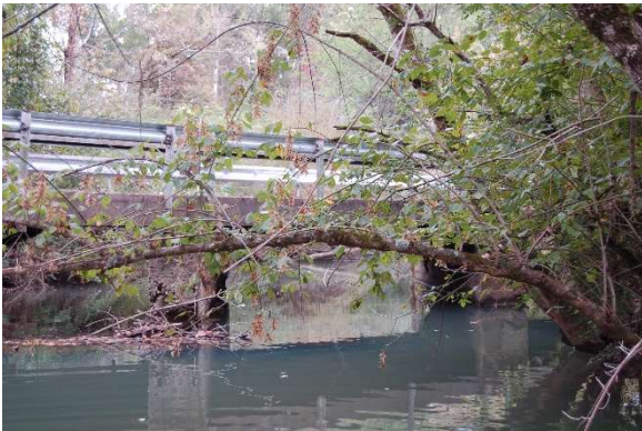
16. Gaines Loop Road Bridge looking downstream
