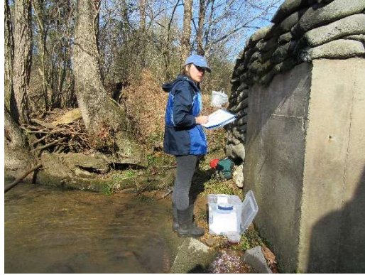
28. Buttrum Road Bridge tributary right bank
