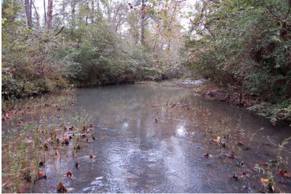
10. Minshew Road Bridge looking upstream
