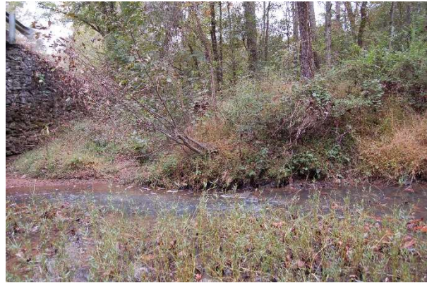
11. Minshew Road Bridge right bank
