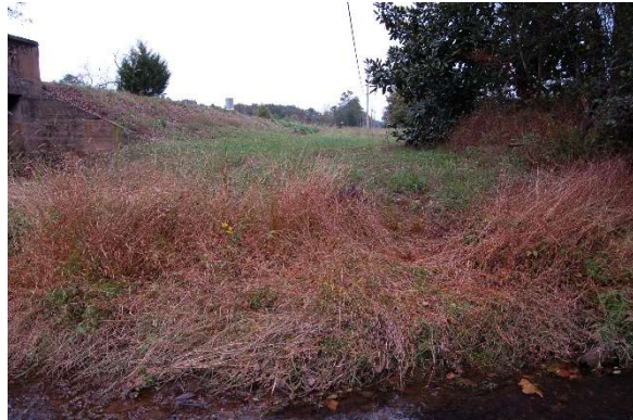
21. Plainville Road Bridge left bank
