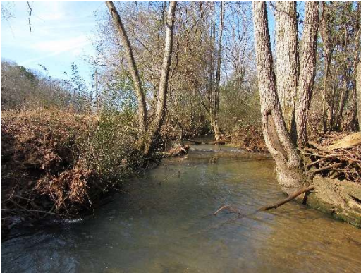
29. Buttrum Road Bridge tributary looking downstream
