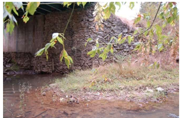
4. Bell's Ferry Road Bridge looking at left bank
