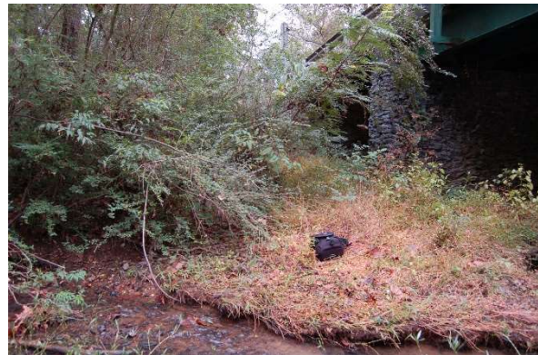
13. Minshew Road Bridge left bank
