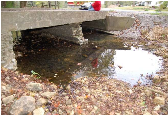
24. Autry Road Bridge looking downstream of site
