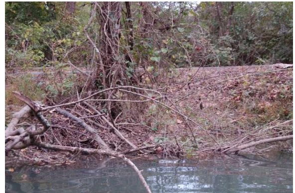
17. Gaines Loop Road Bridge left bank
