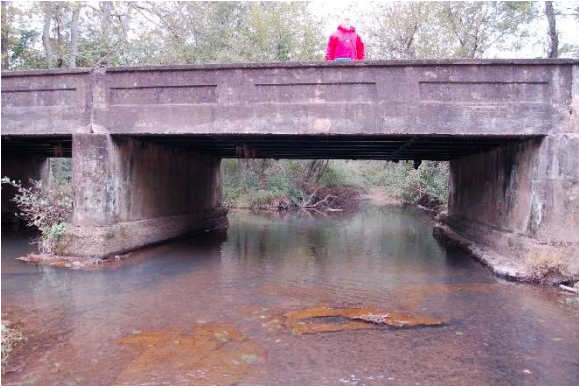
18. Plainville Road Bridge looking upstream
