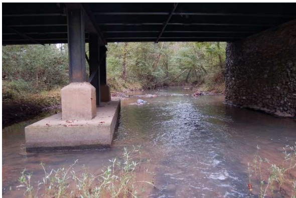
12. Minshew Road Bridge looking downstream
