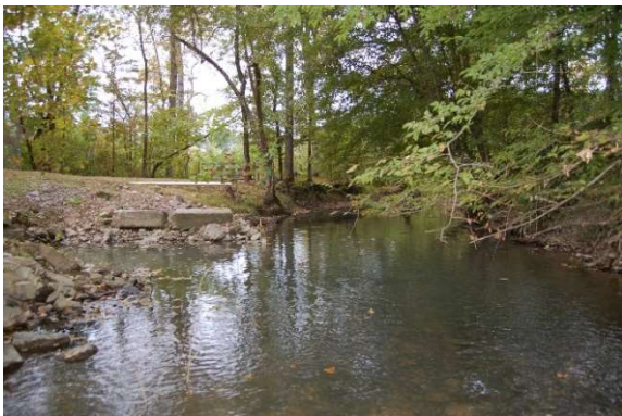
8. Shannon Water intake looking downstream
