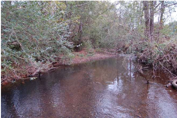
20. Plainville Road Bridge looking downstream
