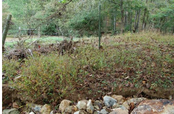
23. Autry Road Bridge right bank
