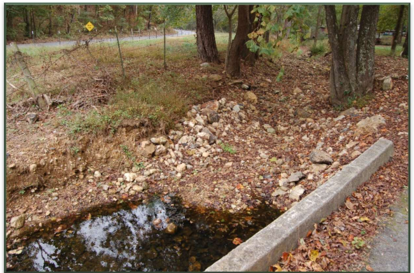
Figure 5. Woodward Creek dry streambed upstream of Autry Road Bridge in October 2018
