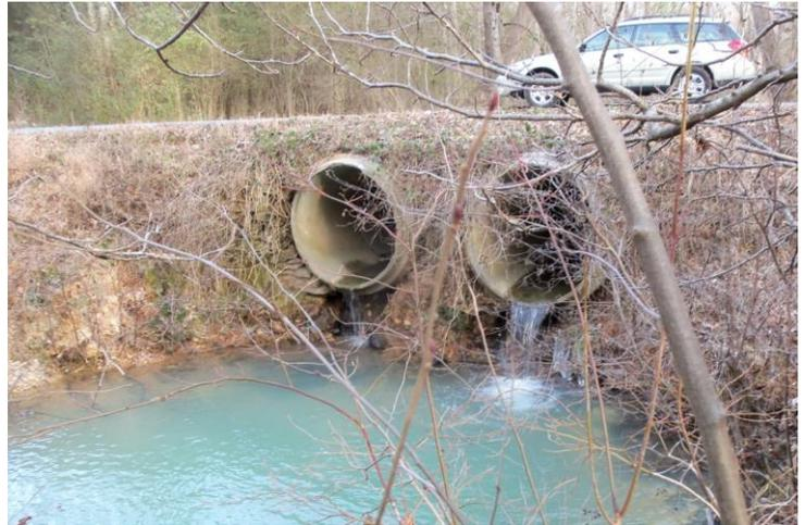
*Figure 3.4. Overshot, failed culvert on E. Hermitage Road. Note the milky appearance of the water.*
